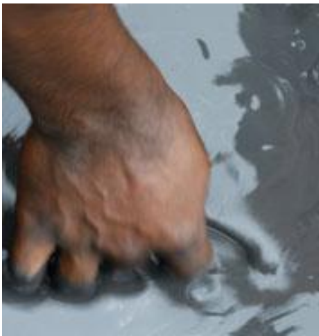
PLATE 3.54: Coating with slurry
